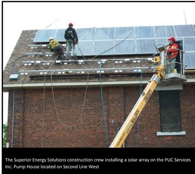
The Superior Energy Solutions construction crew installing a solar array on the PUC Services Inc. Pump House located on Second Line West
